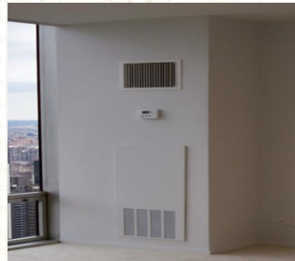
Above, a newly installed HVAC unit
