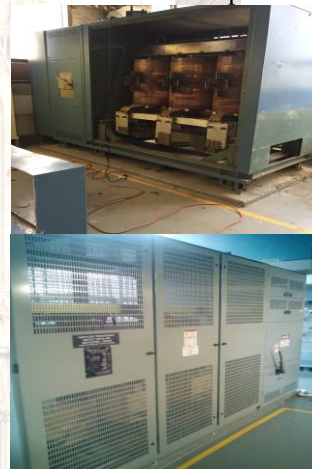
Above: Original Transformer. Below: Newly Installed Transformer
